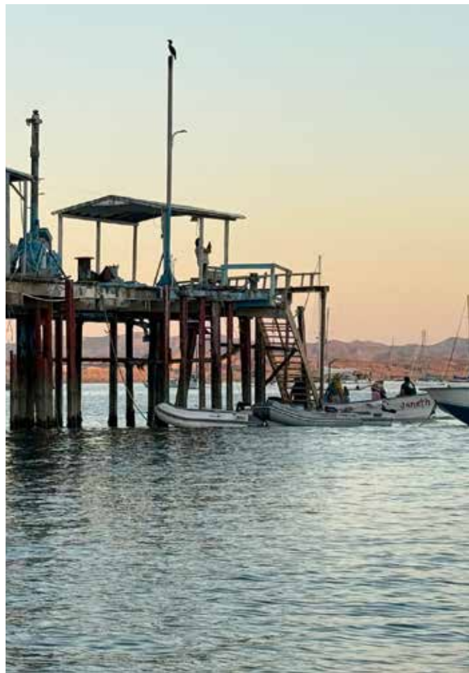
The Turtle Bay pier. The brave stern-tie here and catch the fuel hose from above. Most boats have fuel delivered by panga right to the boat.
